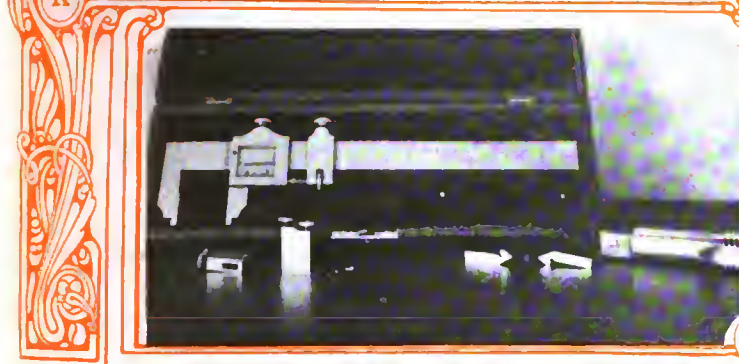
G—Surface gauge on the platen of a Brown & Sharpe No. 4B milling machine.
